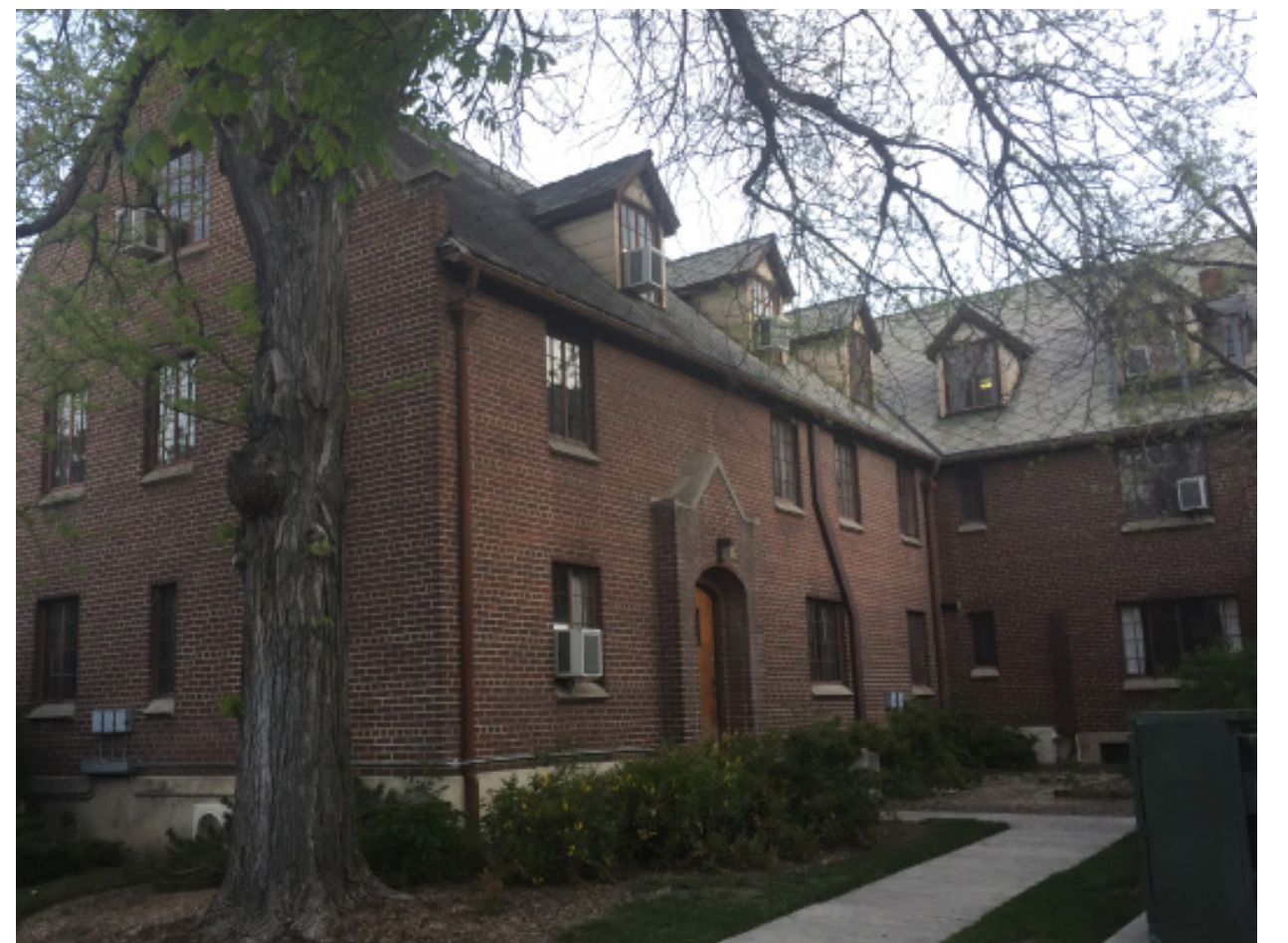
Courtyard Building Small Provo
